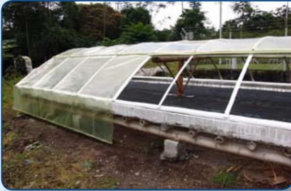
**Figura 4.** Compuertas o tapas laterales enrollables
